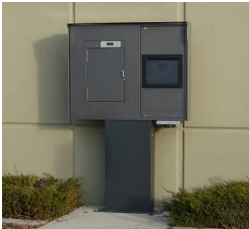
Outdoor enclosure with AC and heater
